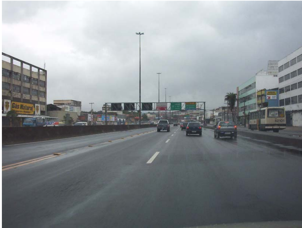
Avenida Brasil (Fully Grade Separated): Entrance to Centro from North 4 Roadways (2 Express, 2 Local): 12 to 14 Lanes One Lane in Each Express Roadway is Busway This is a Secondary Road: Linha Vermelha (Motorway) is Nearby to the East
