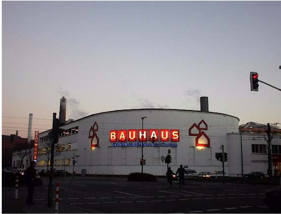
DIY (Home Improvement) Store
