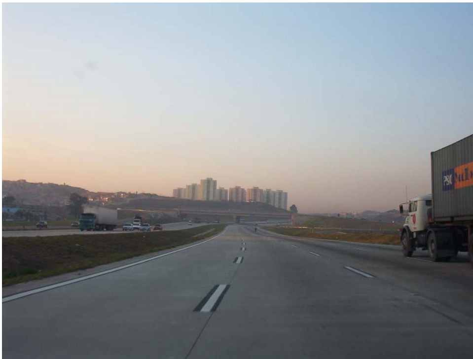
Quarter-Completed Ring Road (Rodoanel Mario Covas)
