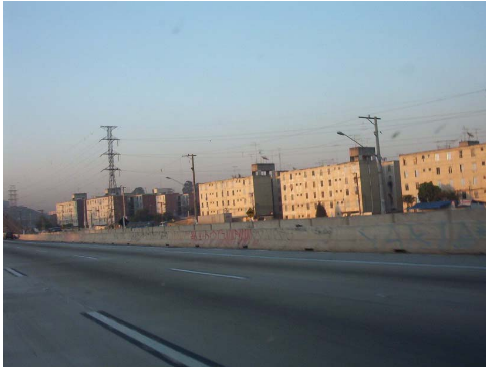
Chicago-Style Favela Replacement High-Rises Adjacent to Ring Road
