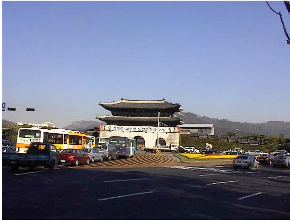
Traditional Architecture in Central Business District
